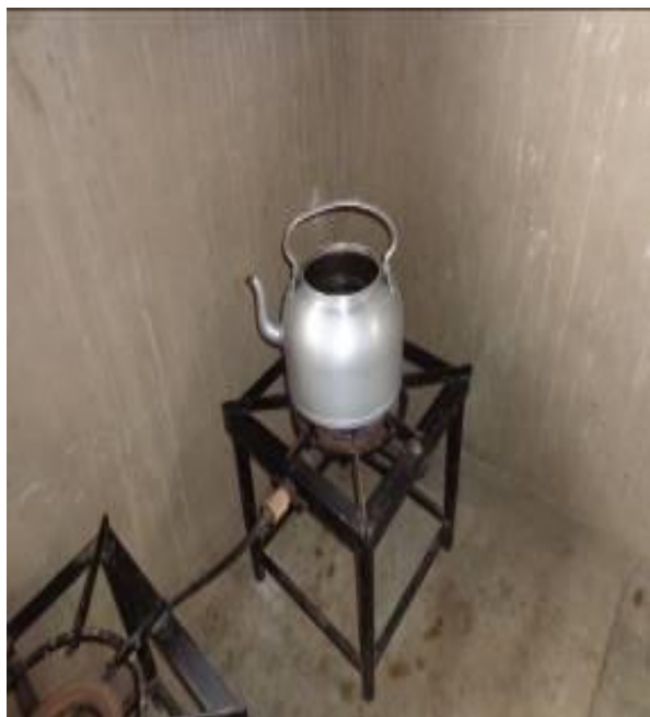
The stoves using biogas tapped from the school latrines
